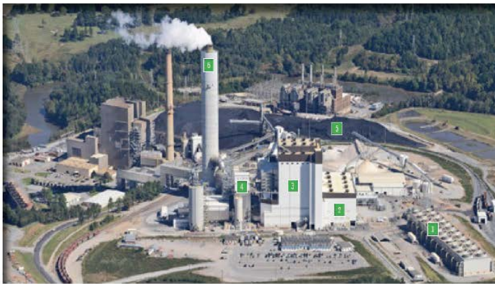
Figure 9.1-15 Illustration of Coal-fired Boiler Control System Configuration Used to Eliminate Wastewater Discharge 29
