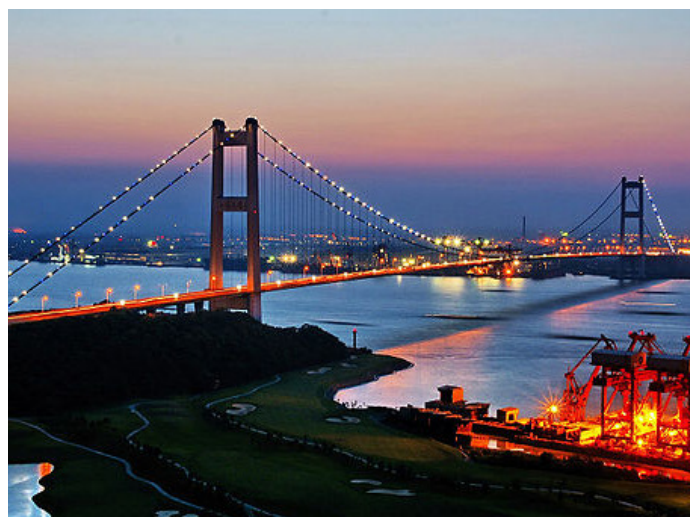
Figure 3-4 Jiangyin Yangtze River Bridge 2
