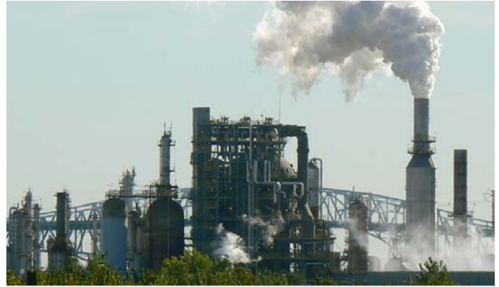
Figure 9.2-3 Photograph of BELCO EDV Wet Scrubber Controlling FCCU Regenerator Emissions 32
