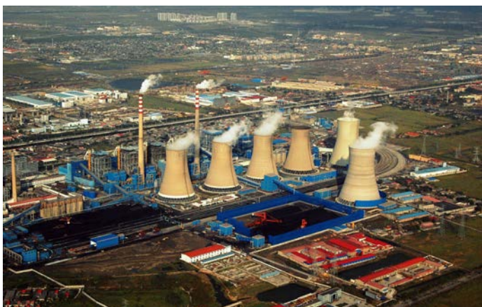
Figure 9.1-8 Photo of Modern Coal-fired Power Plant in China 21
